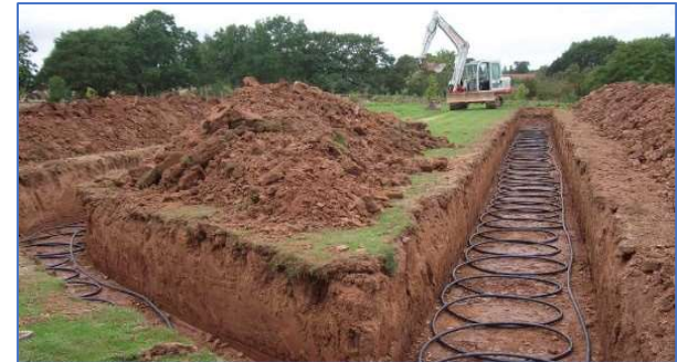
Installation of Ground Source Heat Loops
