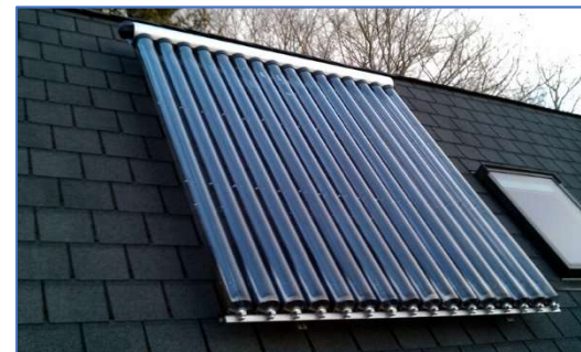
Evacuated Tube Solar Thermal Panel
