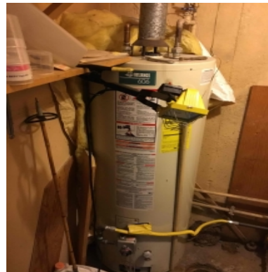
Standard gas water heater.
